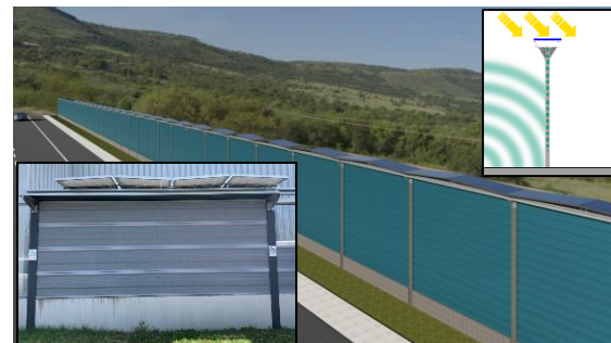
Figure 3: Top-mount solution: Rendering, principle illustration (© ISE) and photo of demonstrator at company R. Kohlhauser GmbH
